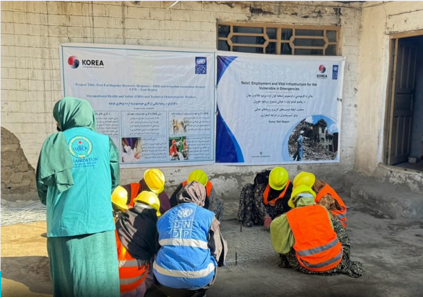
Women working on gabion fence Preparation under the Cash-for-Work program.
