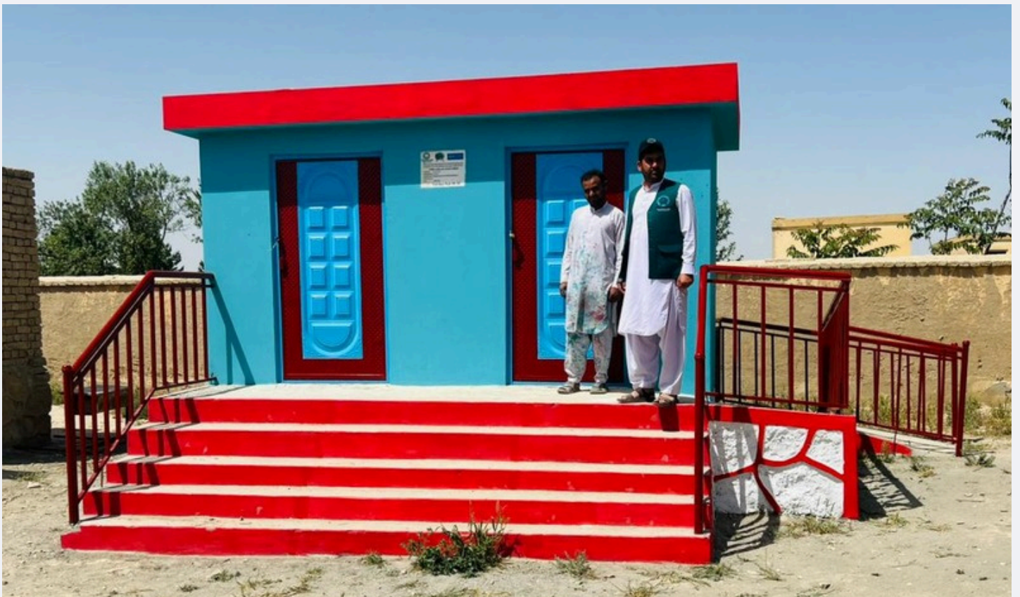
This Photo shows a newly constructed household laterine
