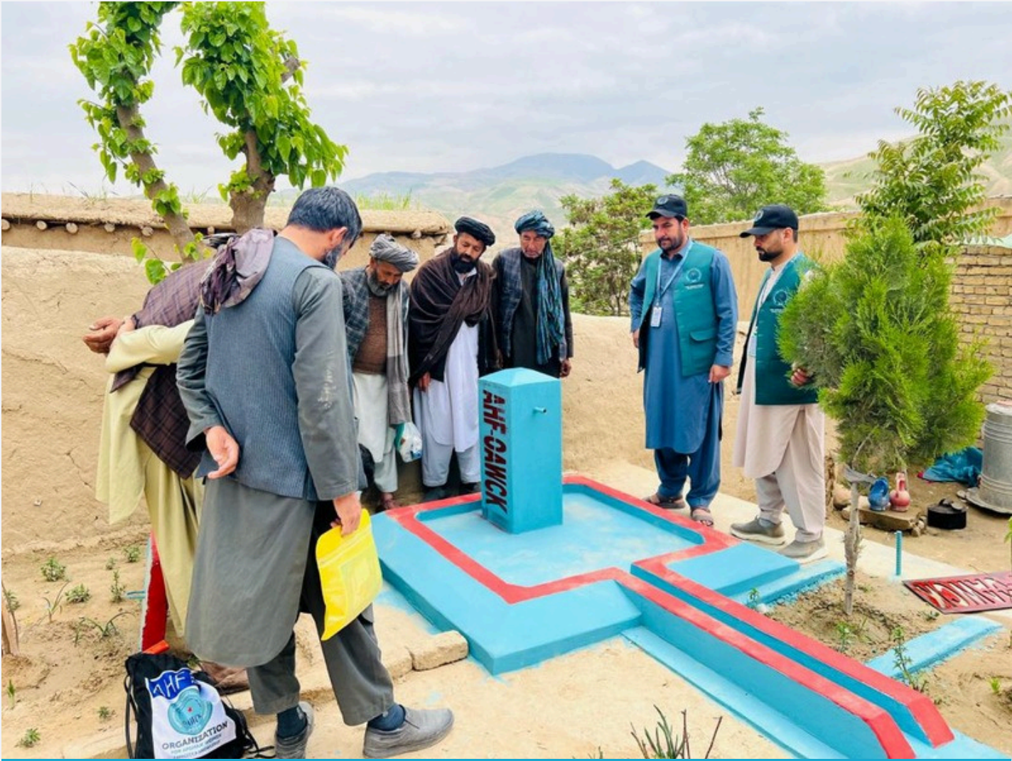
Solar Powered water System, Constructed in Dawlat Abad District, Balkh Province
